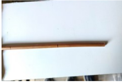
FIG. 6 Marking the copper tube for cutting
